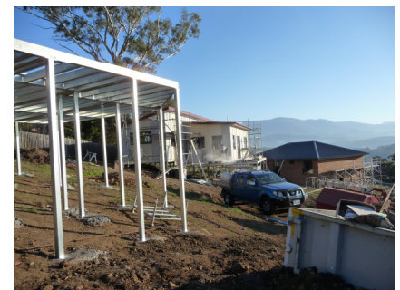
Above: A Quick Build construction site at Mornington.
